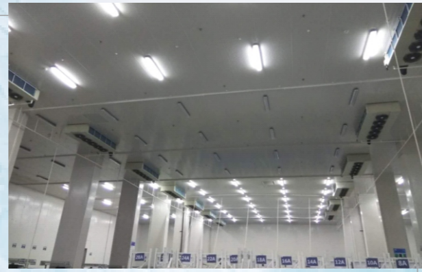
▲ 6,000 square meters of low-temperature storage with a storage height of 8.7 meters (-20°C)
